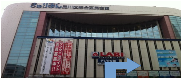
You will find a guideboard in front of the building "Curian" Go to the right side for "the Small Hall".
